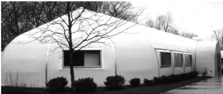
**This tensile structure was built and occupied in 28 days by bioinformatics scientists, who considered it a first-class work environment. When the team disbands or outgrows the space, the structure can be relocated, sold, or stored.**
